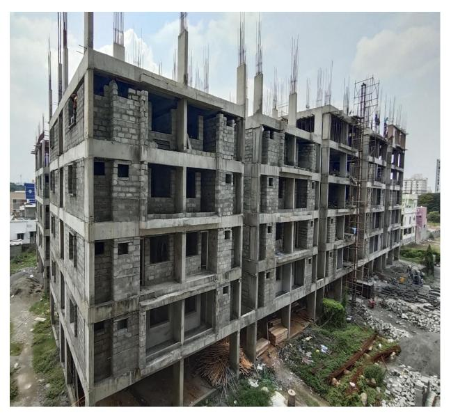
**Block A2:** Fifth Floor Level slab 1<sup>st</sup> half concrete casting 100% completed. Fifth floor Columns concrete 50% completed.
