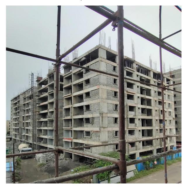
**Block D2:** Terrace Parapet Columns concrete 100% completed. External Plastering work in West side elevation 75% completed.
