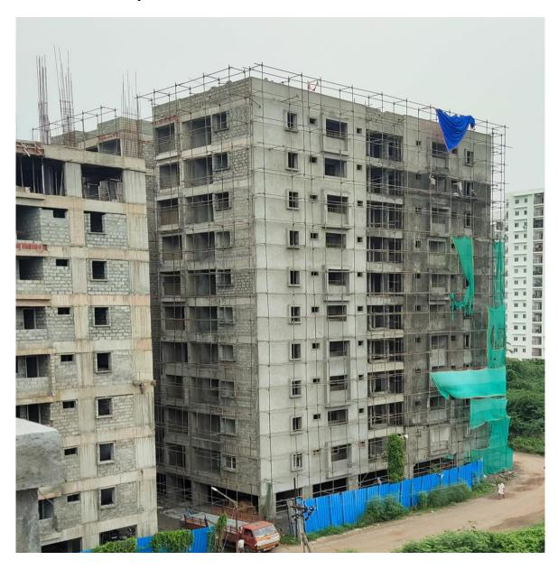
**Block D3: Terrace** Floor level slab 1<sup>st</sup> Half Concrete casting 100% completed. Shuttering & Barbending works for 2<sup>nd</sup> half of Terrace floor level slab on progress.
