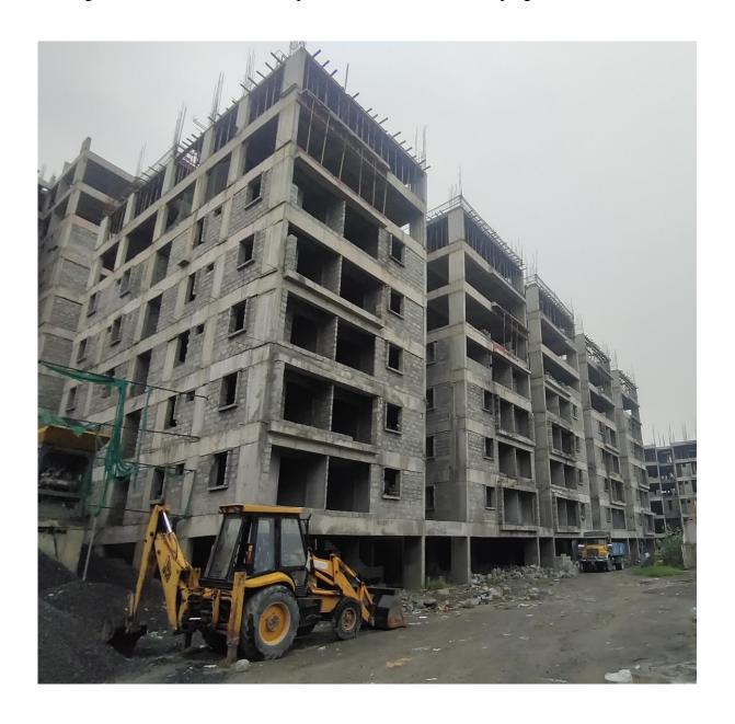
**Block D1:** Ninth Floor level slab 1<sup>st</sup> Half Concrete casting 100% completed. Shuttering works for 2<sup>nd</sup> half of Ninth floor level slab 15% completed.
