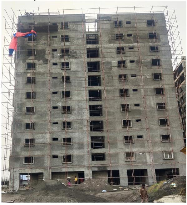
**Block C2:** Terrace floor level slab 100% completed. Parapet Column concrete 90% completed.
